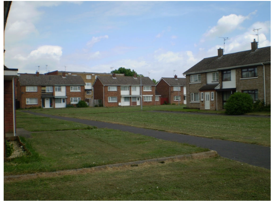
Lack of “defensible space”
