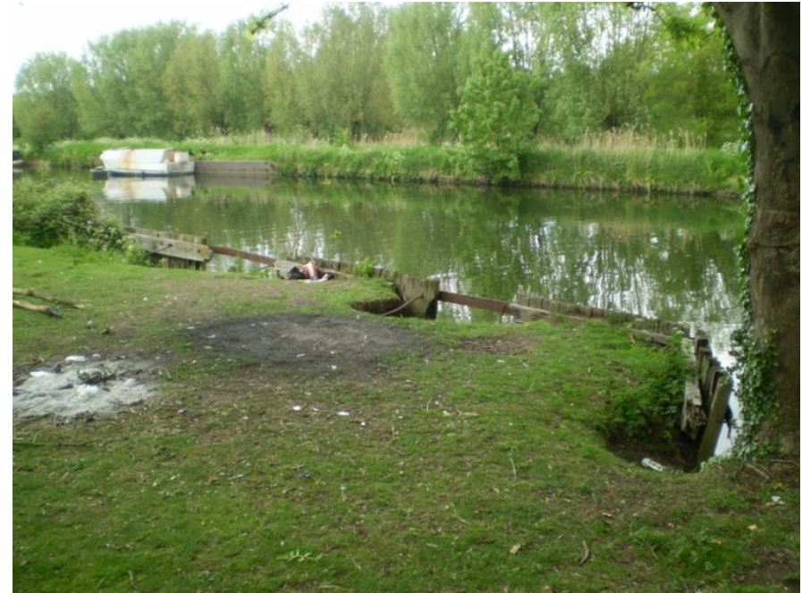
Woodston Wharf (foreground) and abutments to 1901 footbridge and sluice (background)
